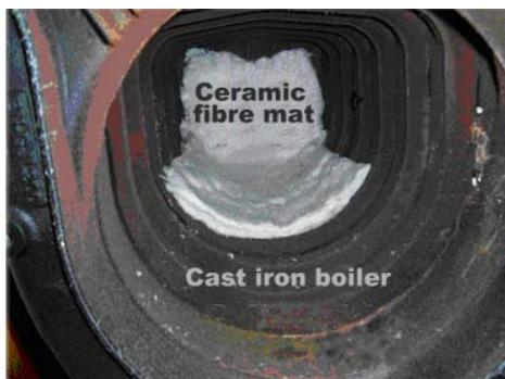
The ceramic fibre mat must be put at the rear end of each cast iron boiler.
